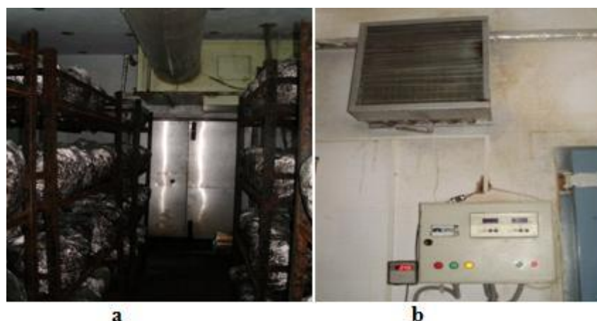
Fig. 6.14 & 6.15 Showing the compost bags kept on shelves for spawn run, the air duct and the Air Handling Unit in the cropping room (a)
